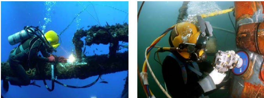
Fig. 1. Typical offshore diving operations: pipeline welding (left) and abrasive cleaning (right). Source: Professional Diving Academy and US Navy.
