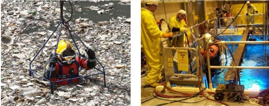
Fig. 2. Hazardous material diving activities: sewage diving (left) and nuclear diving in power reactors (right). Source: NEDCON International LLC.
